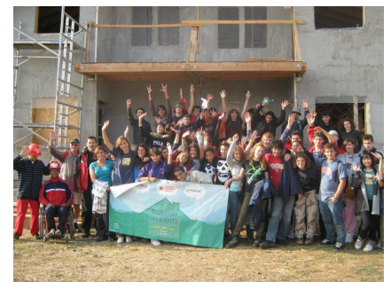
Young people on the construction site in Clinceni
